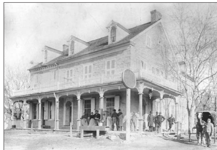
Bowers Hotel was built in 1820 and with the coming of the railroad was enlarged in 1859. This photo is from the late 1800s.
